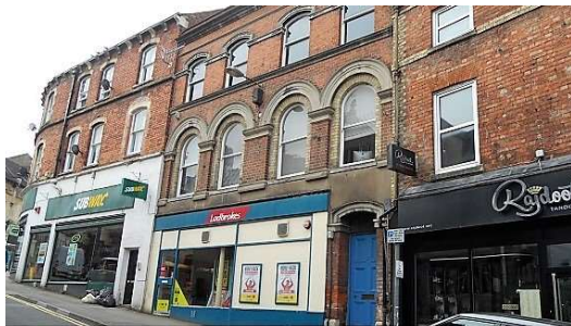
RENT REVIEW COMPLETED STROUD | GLOUCESTER STREET
